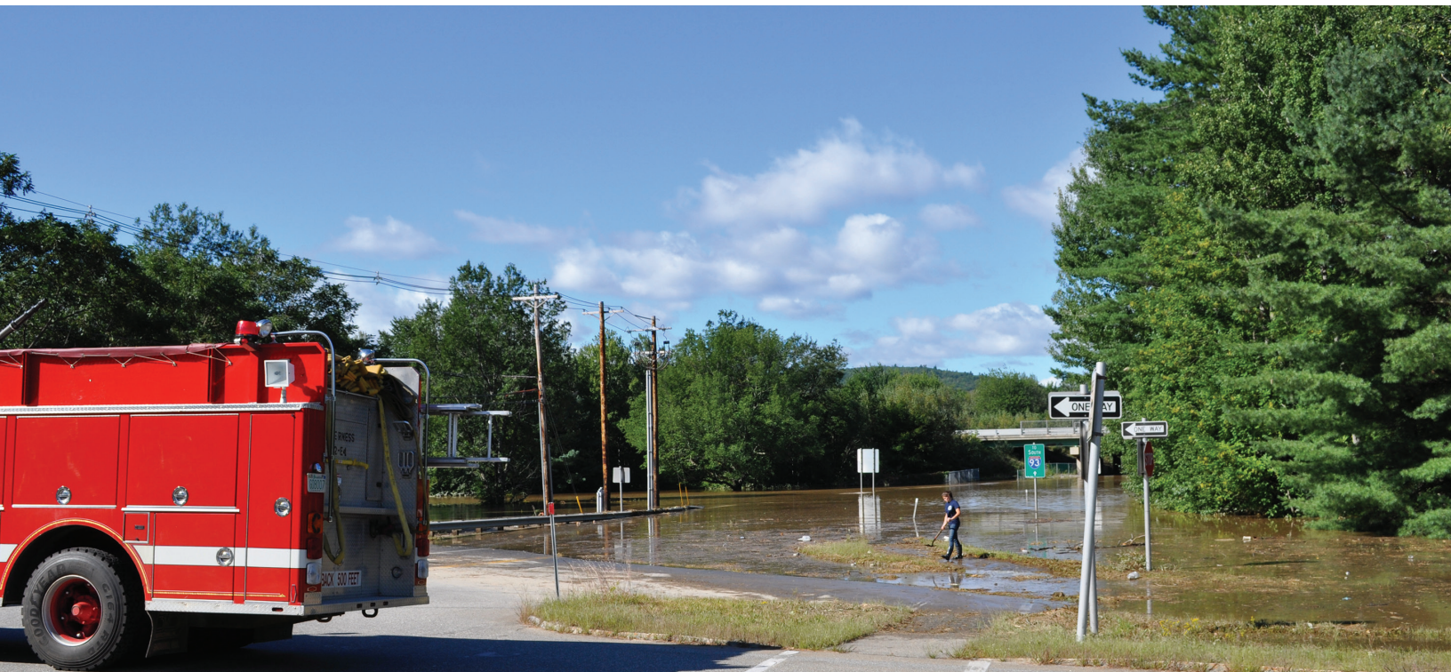
The Pemigewasset River floods after Hurricane Irene hits Plymouth, NH in August of 2011.
