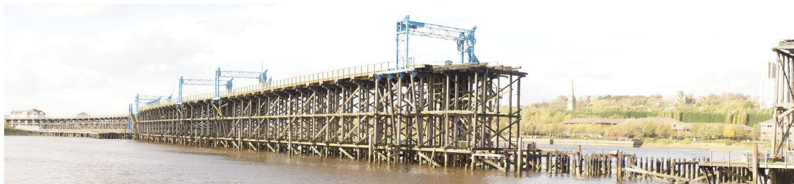
Fig. 1. View of Dunston Staiths, situated on the River Tyne in the northeast of England. (Source: Authors)
