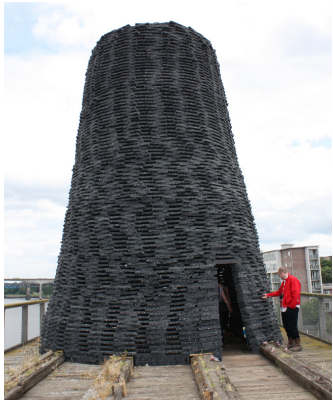
Fig. 2. View of Cone on top of Dunston Staiths, August 2014. (Source: Authors)
