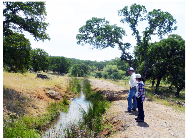
Fig. 3. Water delivery canal. Canals that have not been piped or lined with cement create areas of green riparian vegetation that persists through the dry summers. Water leaking through the earthen floors and walls may provide "return flow," recharging aquifers and emerging lower in the hills in seeps and springs.
