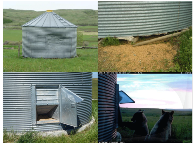
Fig. 7. Examples of grain bin damage caused by grizzly bears ( Ursus arctos ) in our study area. Photo credits clockwise from top left are Andrea Morehouse, Nora Manners, Alberta Environment and Parks/Waterton Biosphere Reserve Association remote trail camera, Spencer Rettler.
