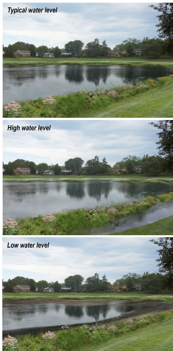
Fig. 1. An example of smart nature-based solutions (sNBS): a retention pond in a residential area that is managed by a smart stormwater system. The pond was depicted with different water levels: (1) typical, (2) low, as if the pond were drained 24 hours before a storm to free up storage capacity, and (3) high, as if water were retained at a higher than typical level for as long as 48 hours after a storm (visualizations by Yiran Shen and Yuanqiu Feng).
