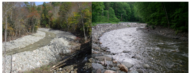
Fig. 3. Chickley River after the channelization; approximately eight km of river were dredged and channelized.
